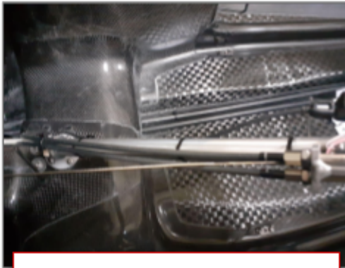
B15.1 Cables must be well secured
